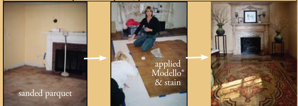
Wood parquet was stained and water damaged-now it's stunning!
