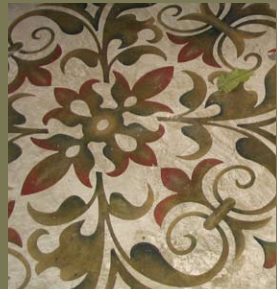
Skimstone was troweled over gray cement floor
