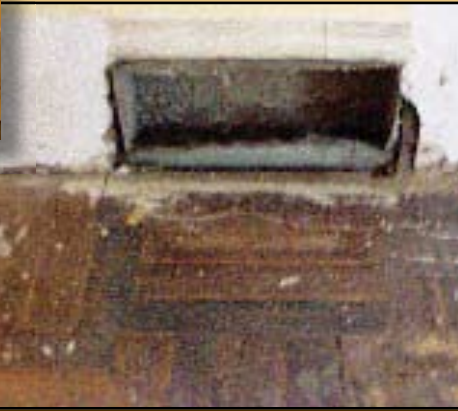
Parquet floor was stained and water damaged
