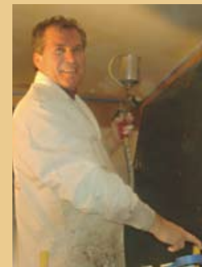
Spraying the ceiling
