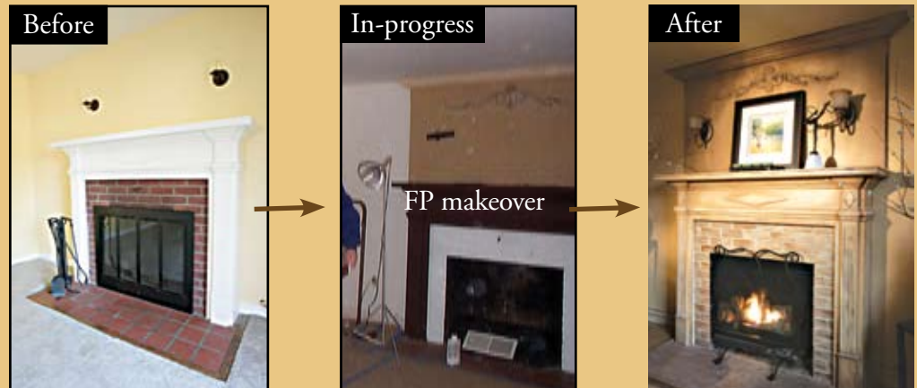
Same fireplace with paint, plaster & MDF board overmantle
