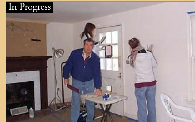
At this stage the walls and brick FP have been primed and wood/trim added above the mantle
