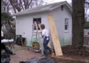
Volunteers primed shed
